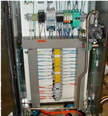
FOUNDATION FIELDBUS CAN SAVE A LOT OF VALUABLE SPACE ON SKID MOUNTED EQUIPMENT
