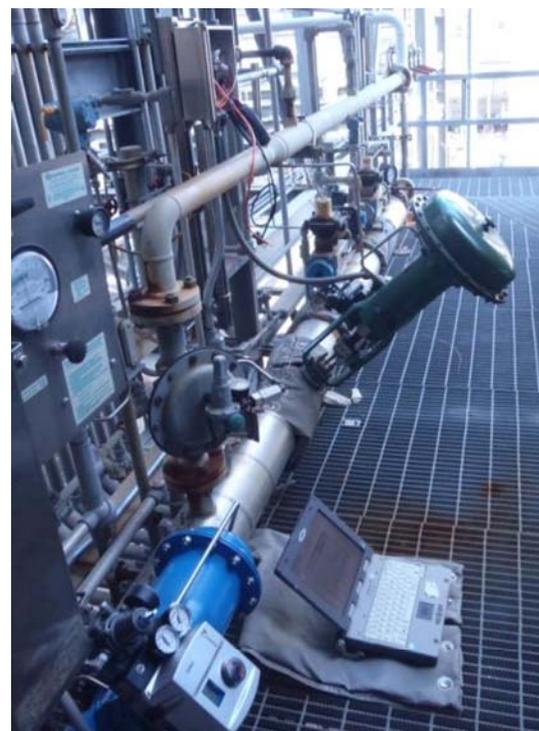
**Remote Wireless Clients can Greatly Simplify the Task of Commissioning Fieldbus Devices Like this Control Valve**
